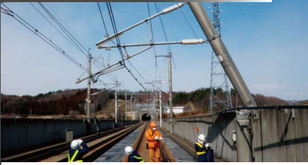
March 2011 Restoration of Tohoku Shinkansen
