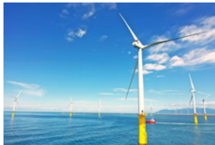
Photo: Akita Offshore Wind Corporation
