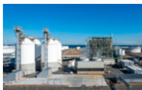
Obayashi Kamisu Biomass Power Plant
