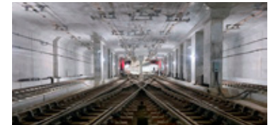
Osaka Station-Tunnel Fukushimahikuzenbashi-Tunnel
