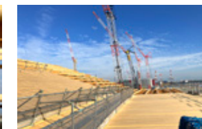
Installing CLT flooring
