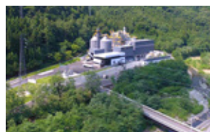
Otsuki Biomass Power Plant (Generating power from Japanese-grown wood)
