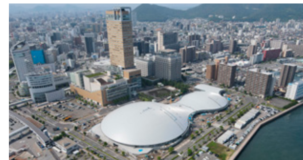
New Kagawa Prefectural Gymnasium (Above: BIM data, Below: Actual construction in progress)
