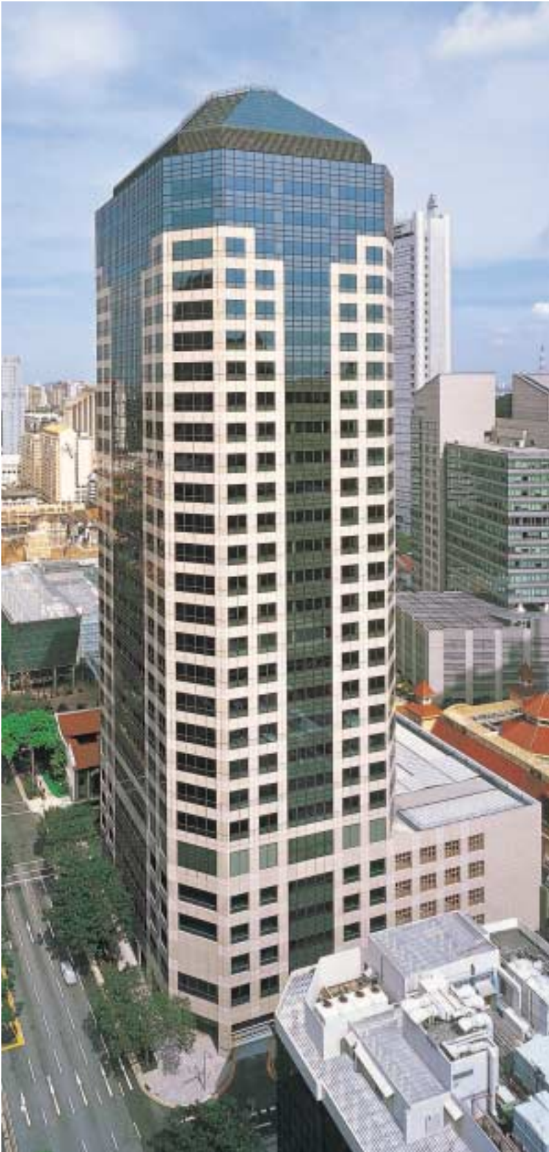
PWC Building (Singapore)
