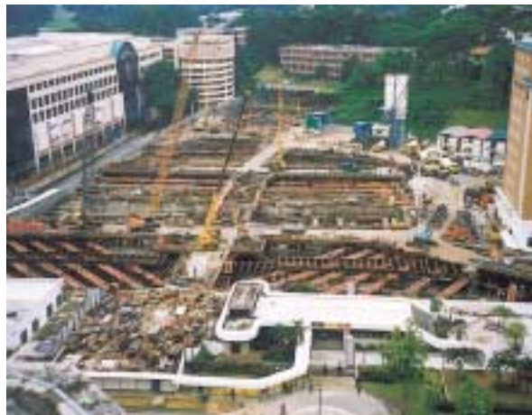
Singapore MRT North-East Line Contract 707 (Singapore)
