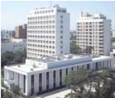
U.S.S.R. Embassy Building
