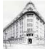
Osaka Shosen Kobe Branch building
