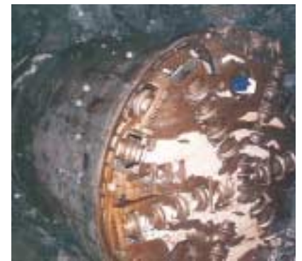
MetroWest Water Supply Tunnel, Contract CP-1 (U.S.A.)
