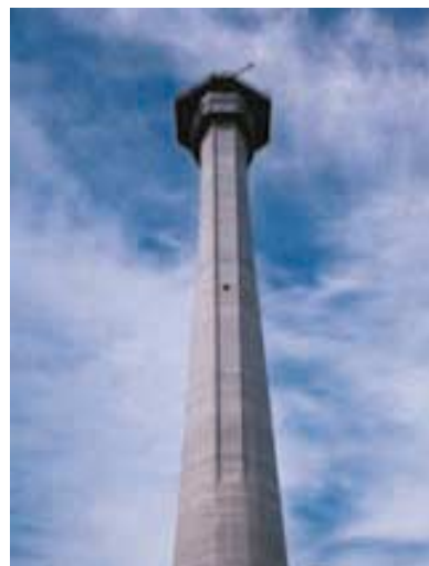
200-meter ultra-high chimney constructed by New Svetho System
