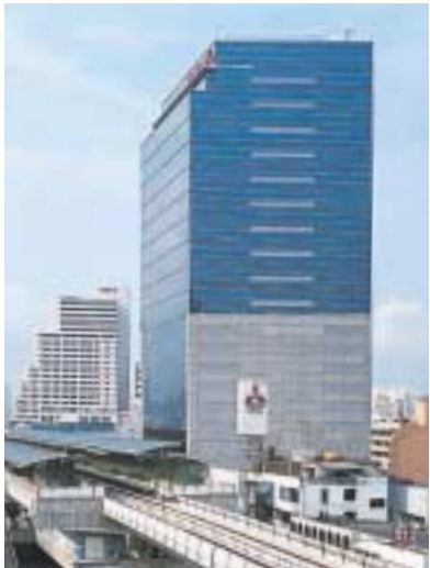
From top: - NEC Computer Storage Philippines, Inc. (Philippines) - School Facilities in Gaza Strip (Palestine) - Sunset Corporate Campus PHASE II (U.S.A.) - Yakult Building (Thailand)
