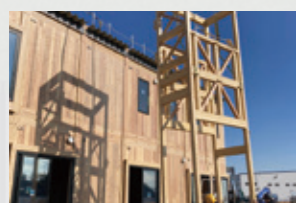
5. Lifting and installing exterior passageway units
