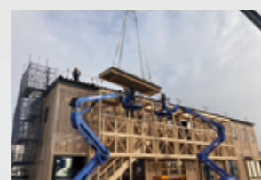
6. Lifting and installing roof units
