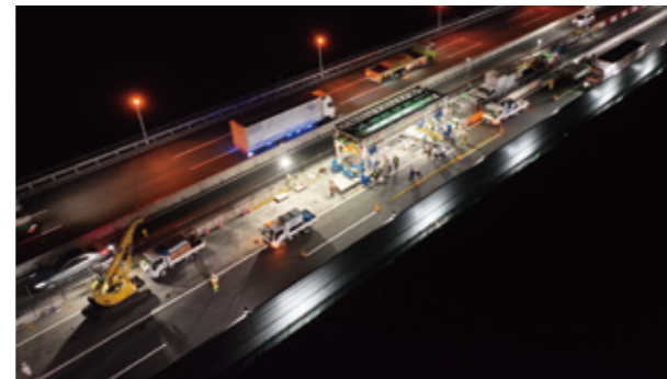
Deck slab replacement using DAYFREE®: Tomei Tamagawa Bridge
