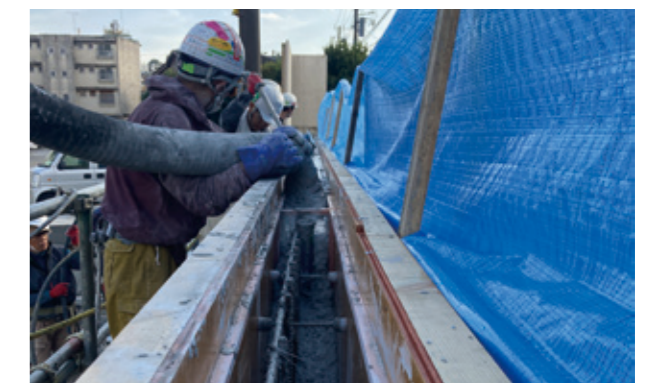
Casting concrete using a concrete pump
