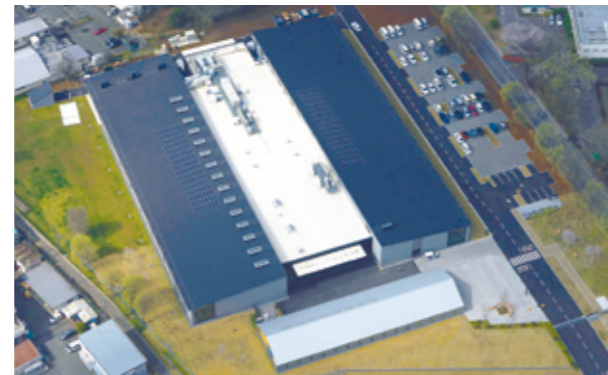
Naigai Technos Corporation's Main Factory
