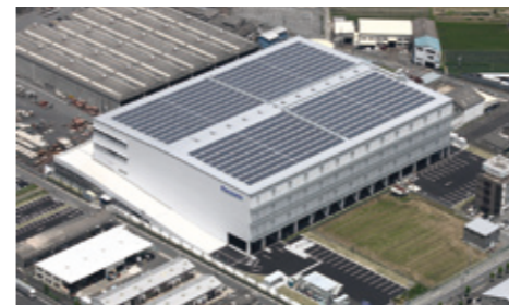
2012 Kumiyama Distribution Center
