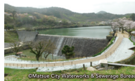
2020 Senbon Dam Reinforcement Work
