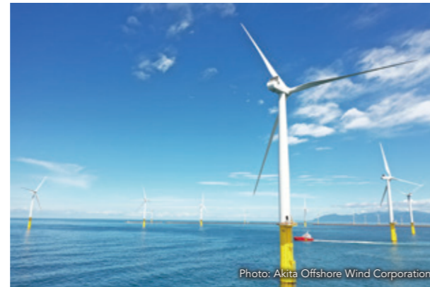
Offshore wind farm at Noshiro Port
