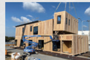
3. Lifting and installing units (second floor)
