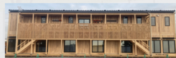
Completed temporary wooden site office
