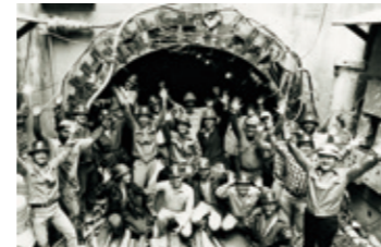
1982 San Francisco Sewer
