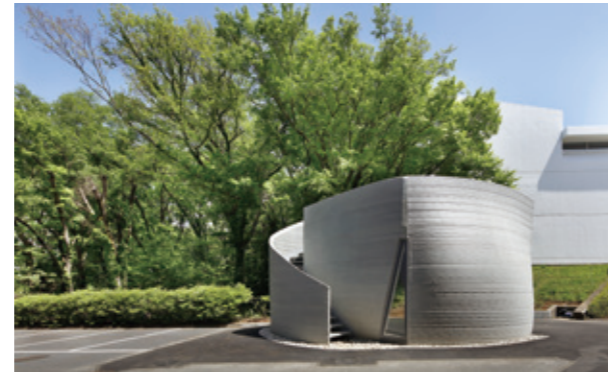
3dpod™, 3D-printer demonstration building https://www.obayashi.co.jp/en/news/detail/news20230425_1_en.html
