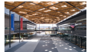
Nara Prefectural Convention Center
