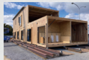
2. Lifting and installing units
