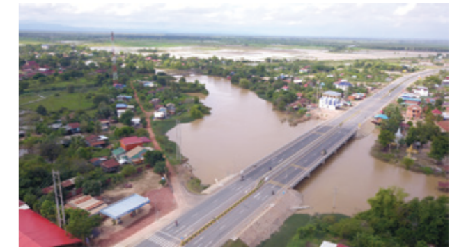
National Road No.5 (Cambodia)
