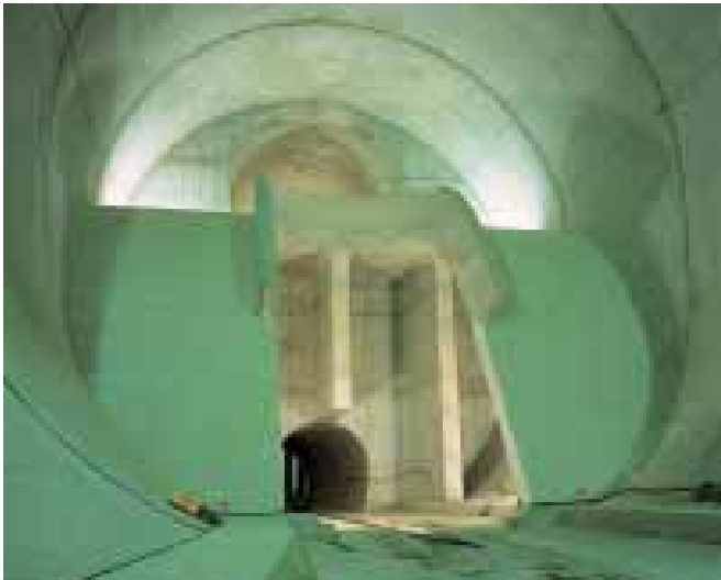
Onmawashi-Koen Regulating Reservoir (Main Tunnel)
