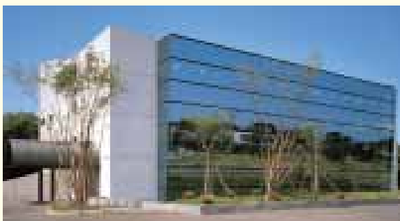
Main Building (Ultra-Energy-Efficient Building)
