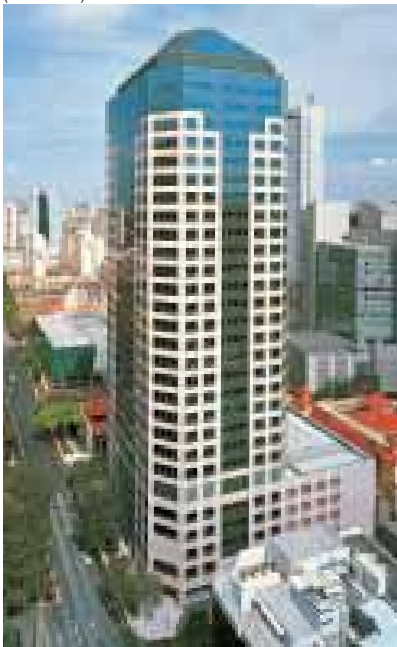
PWC Building (Singapore)
