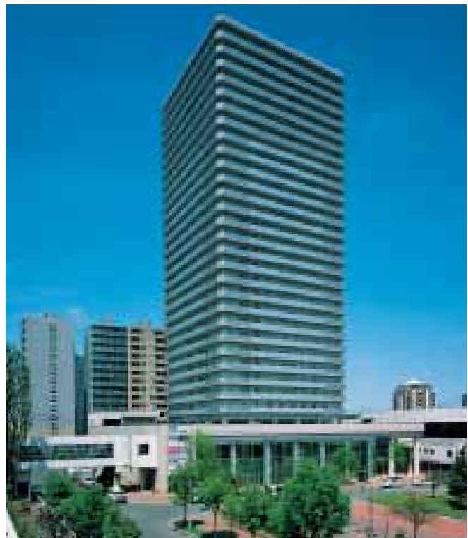
Bellevue Tower Kotoni - Kotoni Tower Plaza
