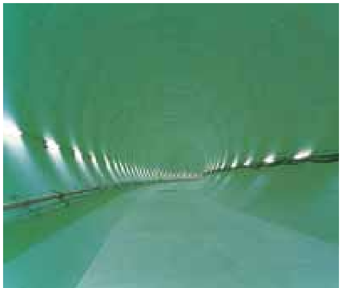
The Metropolitan Area Outer Discharge Channel-Tunnel Contract No.1
