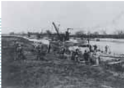
Ocean Landfill Work for Block Yard in the Osaka Port Reconstruction Completed in 1898
