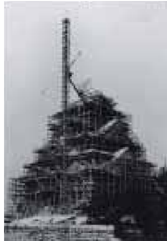
Osaka-jo Castle under renovation Completed in 1931
