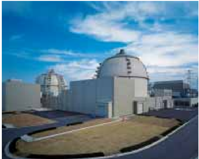
Kyushu Electric Power Co., Inc. Genkai Nuclear Power Station Units 3, 4
