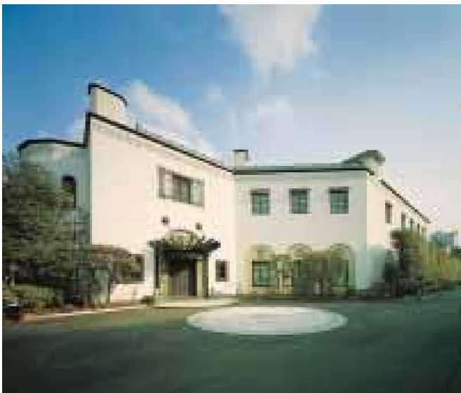
Renovation of the U.S. Ambassador's Residence, U.S. Embassy, Tokyo, Japan
