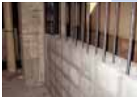
Installation of quake-resistant walls
