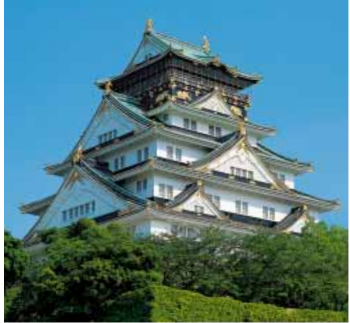
Osaka-jo Castle Tower "The retrofit work of Heisei"
