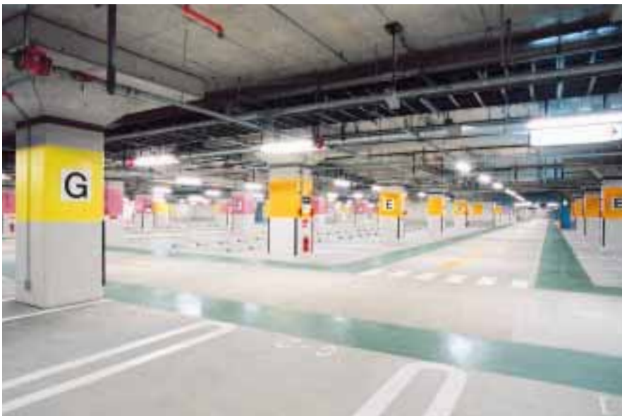
Underground parking (basement level one)
