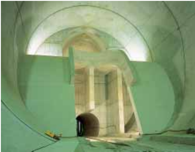
Onmawashi-Koen Regulating Reservoir (Main Tunnel)
