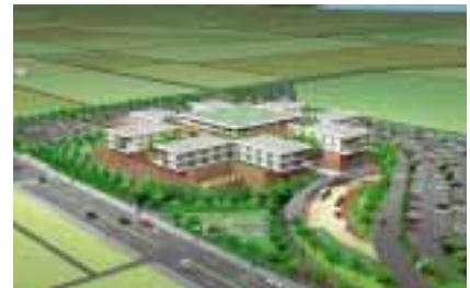
Omihachiman Municipal Hospital Construction and Management Project Omihachiman-shi, Shiga The region's central hospital with 24 examination clinics. Japan's first local government-sponsored hospital of PFI project, with a 30-year BOT method.
