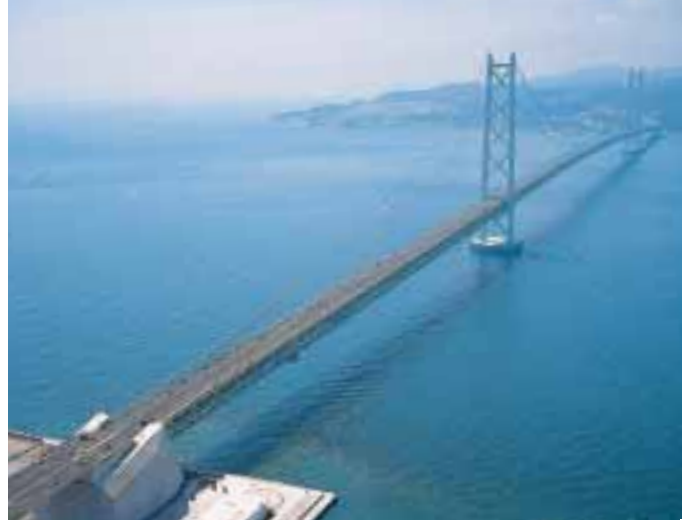
Akashi Kaikyo Bridge (Kobe Side Anchorage)
