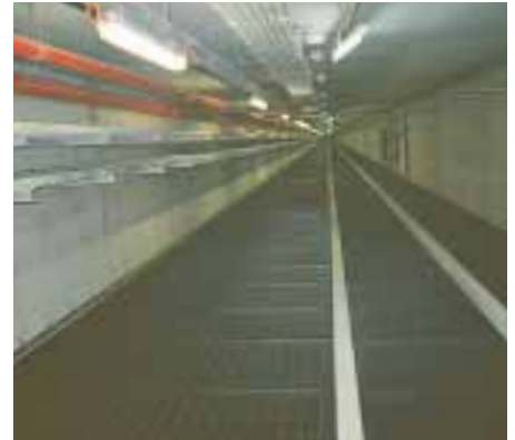
Tuas Immersed Tunnel
