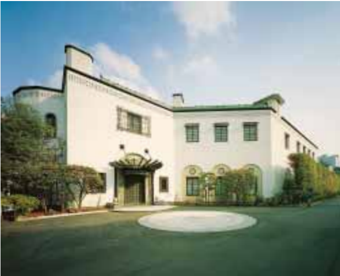
Renovation of the U.S. Ambassador's Residence, U.S. Embassy, Tokyo, Japan
