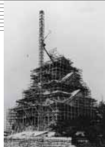
Osaka-jo Castle under renovation Completed in 1931
