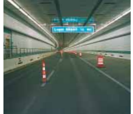
Central Artery/Tunnel, Boston Ted Williams Tunnel C07 A1
