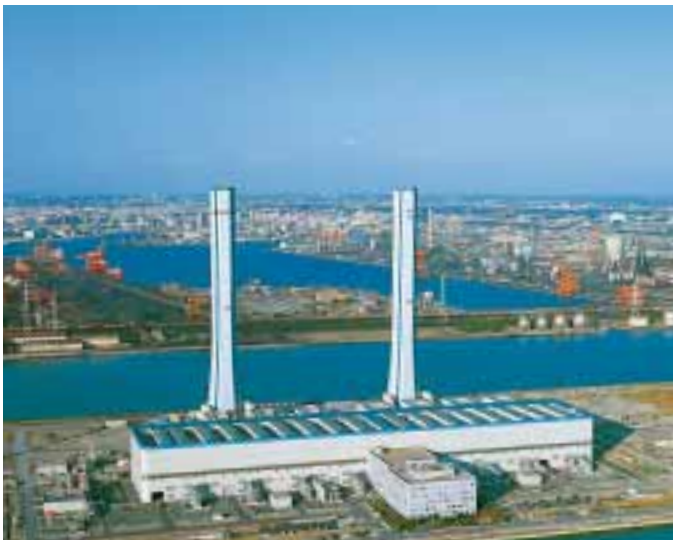
Tokyo Electric Power Co., Inc. Chiba Thermal Power Station
