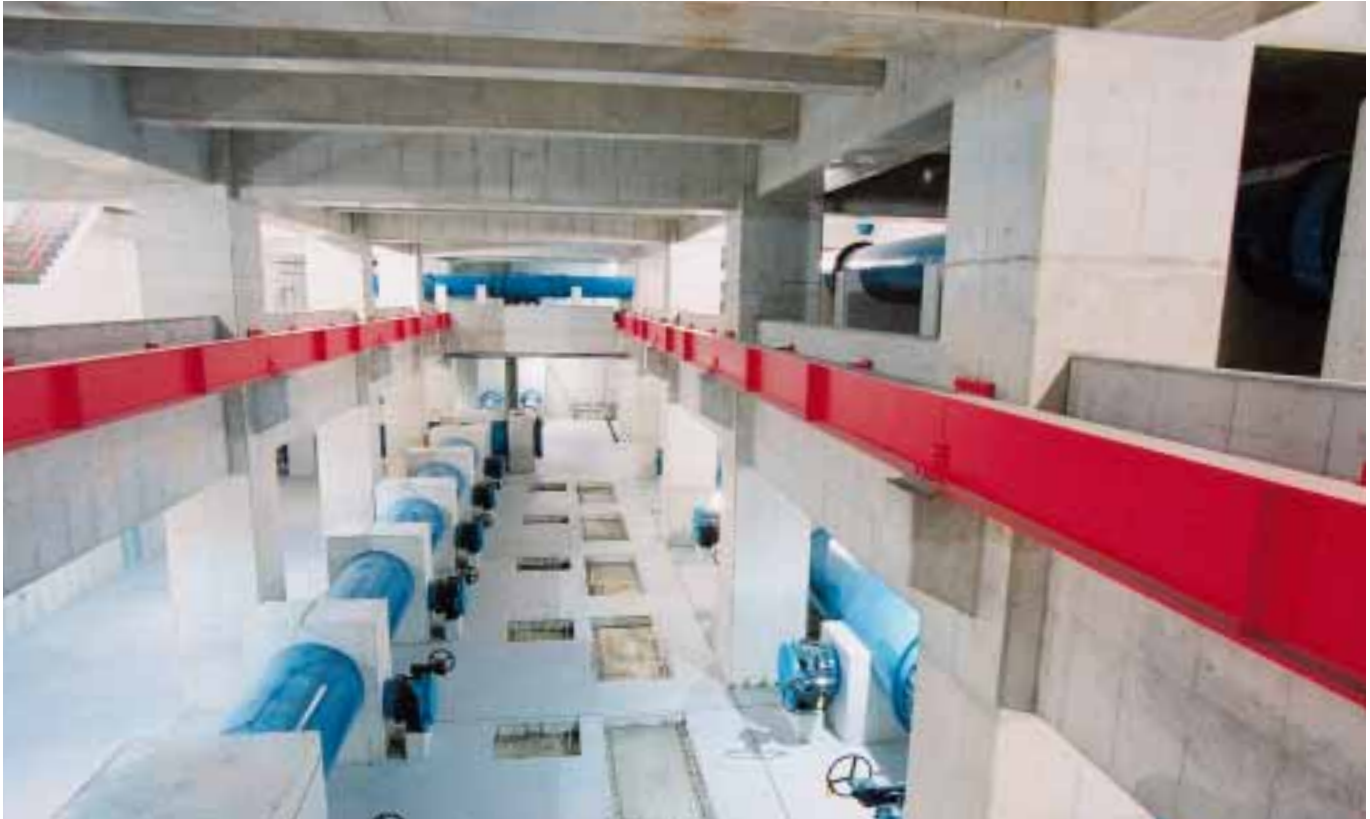
Underground drainage canal (basement level two)
