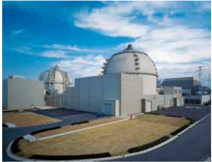
Kyushu Electric Power Co., Inc. Genkai Nuclear Power Station Units 3, 4
