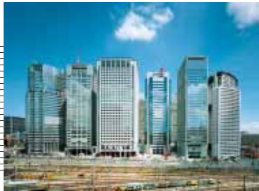
The development area of the JR Shinagawa Station East Exit District As of 2002
