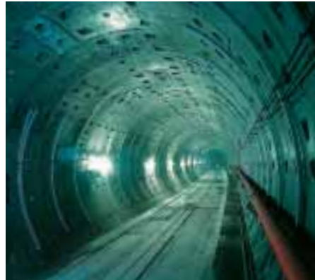
Taipei Metropolitan Area Rapid Transit Systems, Hsintien Line Contract 218
