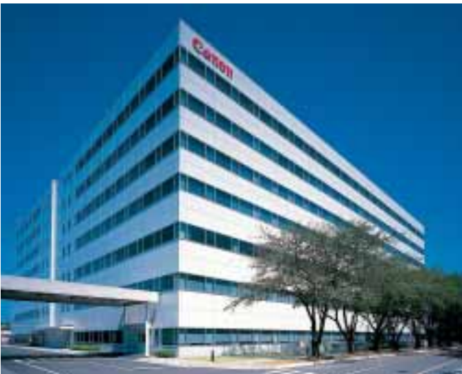
Canon Inc. Toride Plant 98A-B-1 Building
