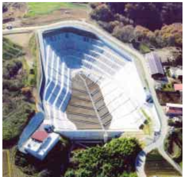
Annaka General Waste Final Processing Plant Location: Gunma
