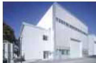
Fire Protection Engineering Laboratory
