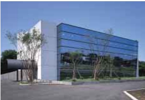
The Main Building (The Super Energy-Conservation Building)
