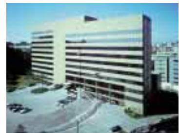
U.S. Embassy Office Building
