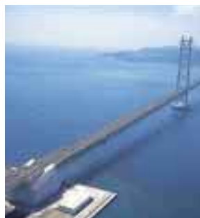
Akashi Kaikyo Bridge (Kobe Side Anchorage)
