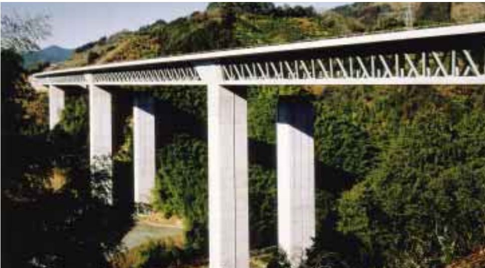
The Second Tomei Expressway Sarutagawa-bridge and Tomoegawa- bridge Location: Shizuoka
