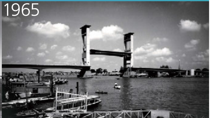
The Musi River Bridge in Indonesia was a pioneering project for us outside Japan.
