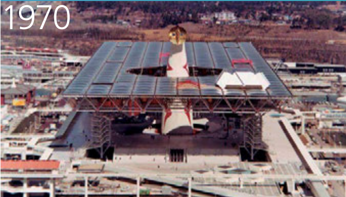
The Big Roof of the Japan World Exposition (Theme Pavilion) used a liftup construction method of an unprecedented scale.
