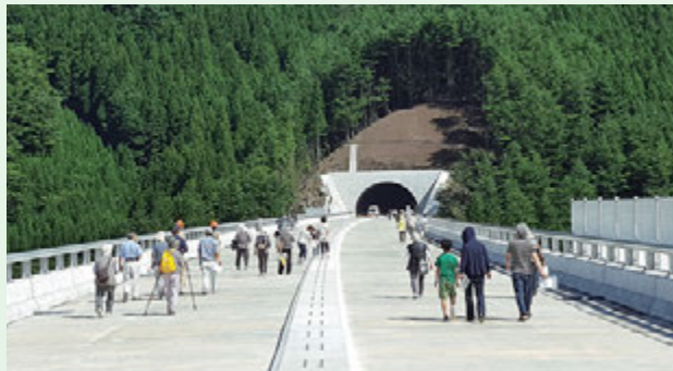
About 1,000 people toured the road over the 3 years and 7 months of the project. The tours expressed the appeal of building things and the attractiveness of the construction industry.
