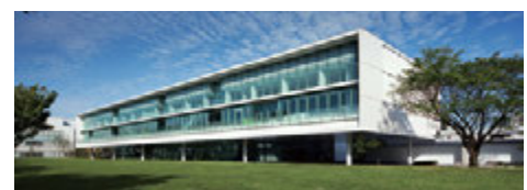
Techno-Station, the main building at Technical Research Institute About 4,000–5,000 customers, students, and others visit annually.
