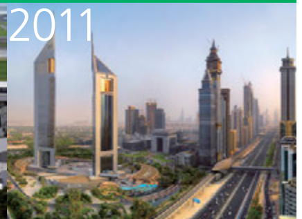
Dubai Metro Project
