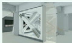
Cross Dampers installed in Kumamoto Castle Main Tower as part of its restoration (installed image)
