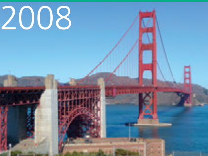
Golden Gate Bridge seismic retrofit
