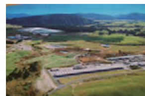
A geothermal power plant operated by Tuaropaki Trust
