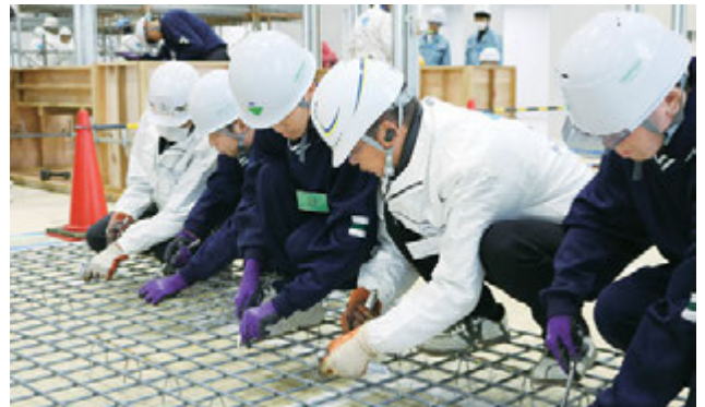
Senior high school students learn how to assemble iron reinforcing bar.
