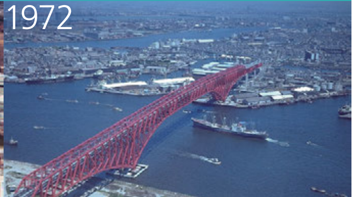
The Minato Bridge on Hanshin Expressway Route 5 Bayshore Line had the longest span of any truss road bridge in Japan when it was completed.
