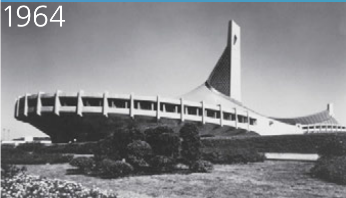
Yoyogi National Stadium 2nd Gymnasium, constructed for the Tokyo Olympics. The curving roof, suspended from cables, is exemplary of Japanese modernist architecture.
