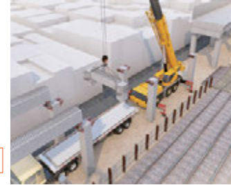
Hokuriku Shinkansen Fukui Development Viaduct construction project This is the first use of precast units on a Shinkansen rigid-frame viaduct (under construction).
