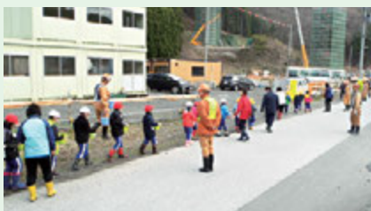
Directing local traffic and cleaning up around construction sites are part of our day-to-day work. At construction sites around Japan, we direct traffic and run patrols daily. Our goal is to ensure the safety of local residents.
