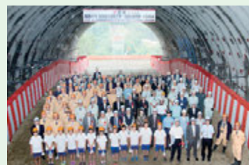
We invited local elementary school students, residents, and the chamber of commerce and industry to the tunnel breakthrough ceremony. During the three years of the project, we kept close to the community.
