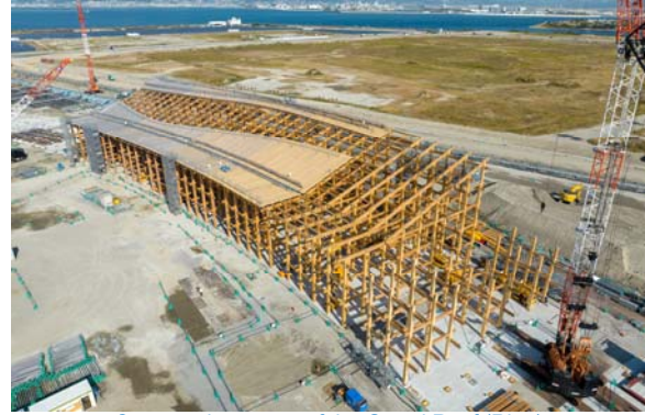
Construction status of the Grand Roof (Ring) at Pavilion World northeast section
