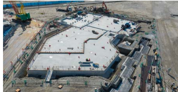
Construction status of Panasonic Group's pavilion
