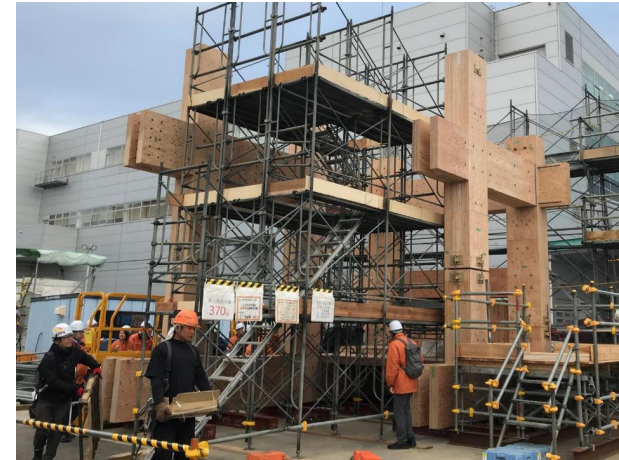
Obayashi Training Center [construction test]
