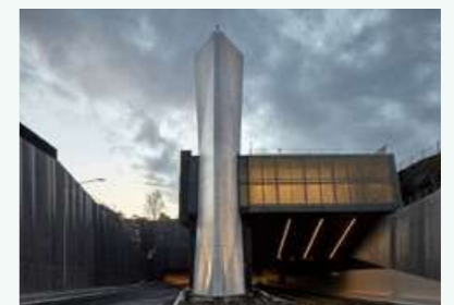
The tunnel's ventilating stack. Ventilation power consumption has been suppressed, saving about 4,600 t-CO 2 per year.
