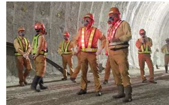
A patrol checking dust hazard prevention efforts in a tunnel
