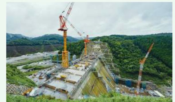
Automatic concrete transportation system using tower cranes
