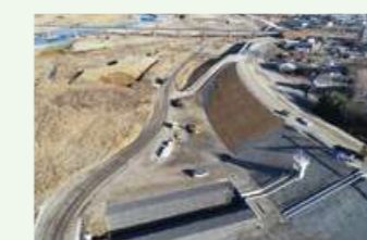
Ground level raising by ICT-based machinery
