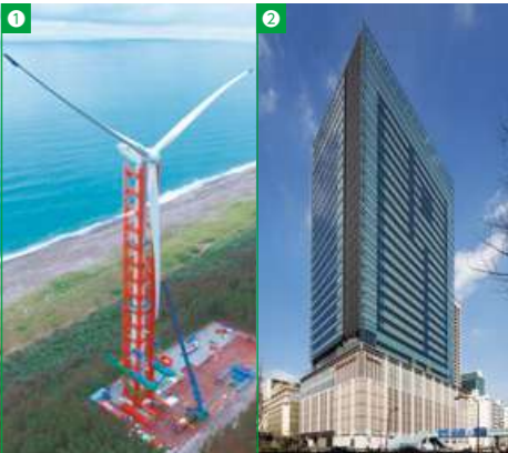
Mitanehamada Wind Power Station Construction Project (the First Construction Excellence Prize) | Nihonbashi 2-Chome Type-1 Urban Area Redevelopment Project (the 61st BCS Prize)
