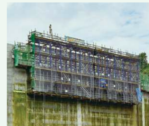
Dam formwork automatic sliding system automates concrete formwork transfer and placement.
