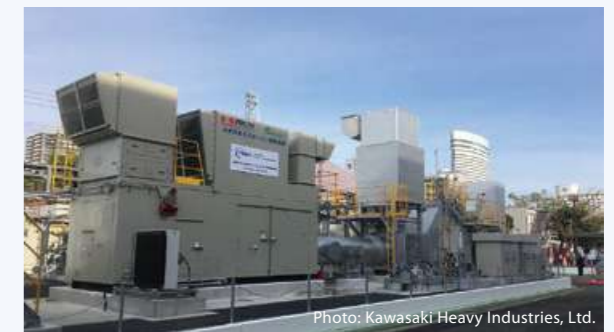
100% hydrogen-fueled gas turbine verification plant with dry low-NOx combustion (a NEDO-subsidized project)
