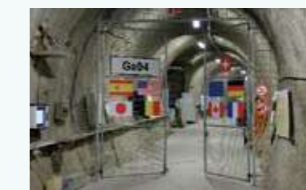
A gate to the experimental area (Gallery Ga04) at the Mont Terri Rock Laboratory. © swisstopo
