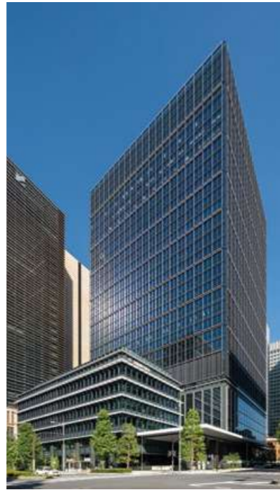
Mizuho Marunouchi Tower, with Japanese Bankers Association Hall in the low-rise portion
