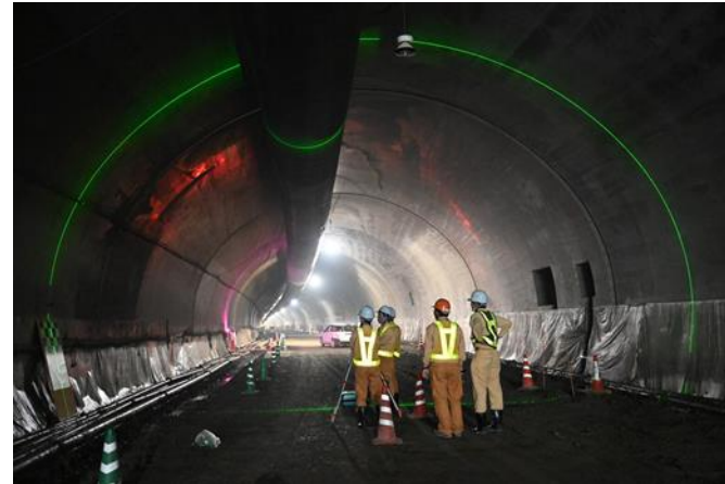
Picture left: On-site measurement
