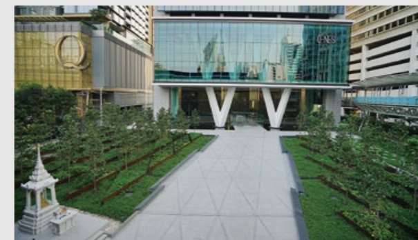
The forecourt design inspired by the shape of V-column harmonizes with the building
