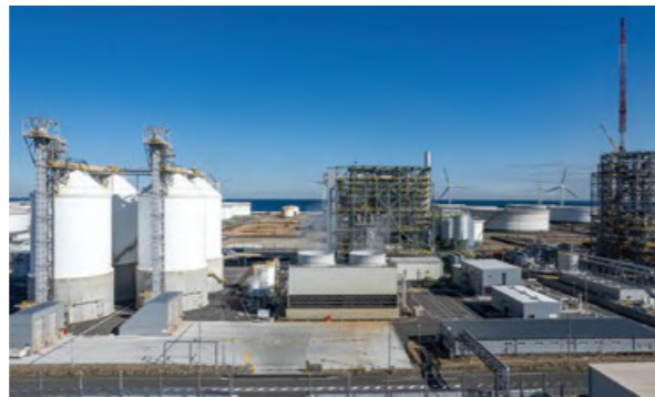
Obayashi Kamisu Biomass Power Plant
