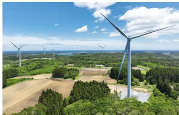
Kamikita-Ogawara Wind Power Station
