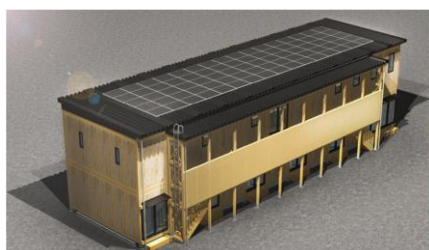
First wooden temporary site office in Japan to receive ZEB certification: Temporary Construction Site Office of Iwatani Corporation New Training Facility
