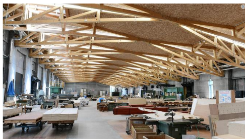
Large-scale plant with hybrid structure of wood and concrete Reconstruction of Naigai Technos head office and factory
