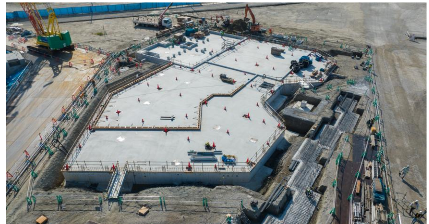
Construction status of Panasonic Group's pavilion
