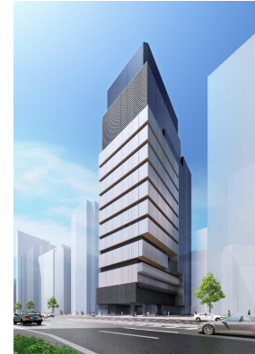
Completed image of the first urban DC to be opened in Minato Ward, Tokyo in FY2028
