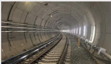
Osaka Metro Chuo Line Yumeshima Station
