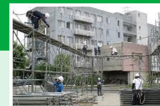
Scaffolding assembly training
