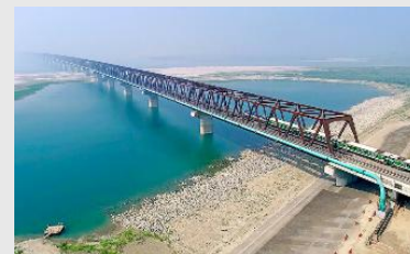
Jamuna Railway Bridge (Eastern Part of Civil Works Package WD-1 / Bangladesh)
