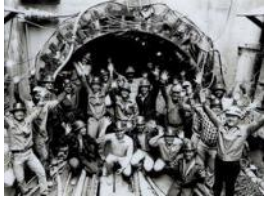
1982 San Francisco Sewer
