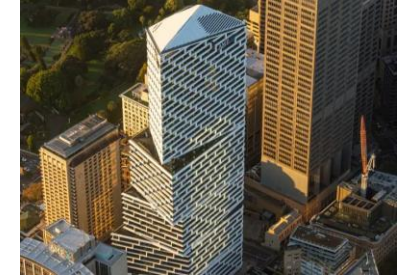
Quay Quarter Tower (Office in Sydney)
