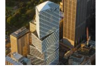
Quay Quarter Tower (Office in Sydney)
