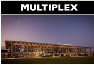
Western Sydney International Airport Terminal (空港、シドニー)
